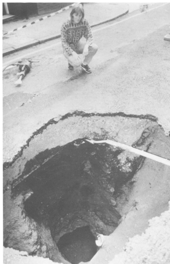
FIG. 3. Crown hole above the failed roof of the Stanford Street cave in June 1990.
