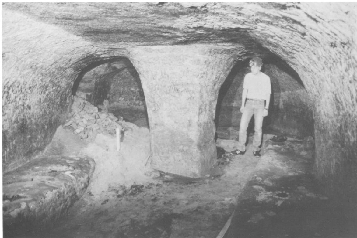
FIG. 1. A typical Nottingham cave—one of the old beer cellars beneath the Corner Pin public house. The flat roof section in front of the rock pillar subsequently failed (see Fig. 7).
