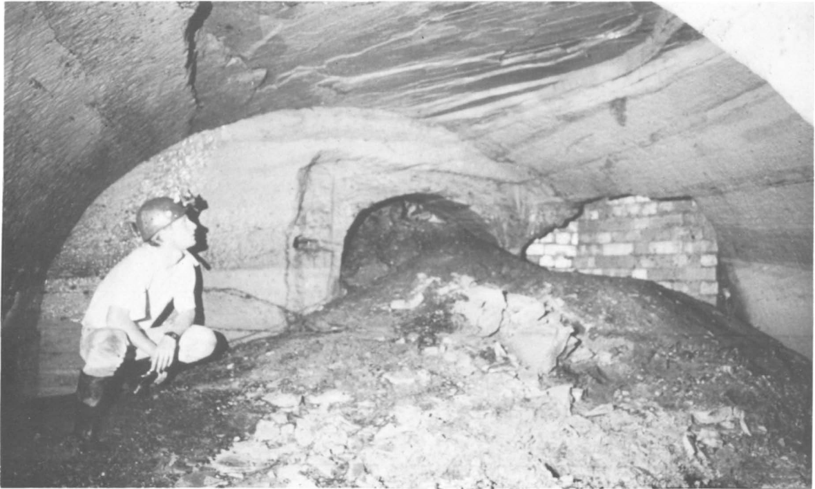
FIG. 6. (above) Saturated sandstone breaking into thin beds and falling away from the roof arch at the southern end of the Stanford Street caves. The light material on the debris pile is fallen roof, some remaining in thin slabs, other broken to sand on impact.
