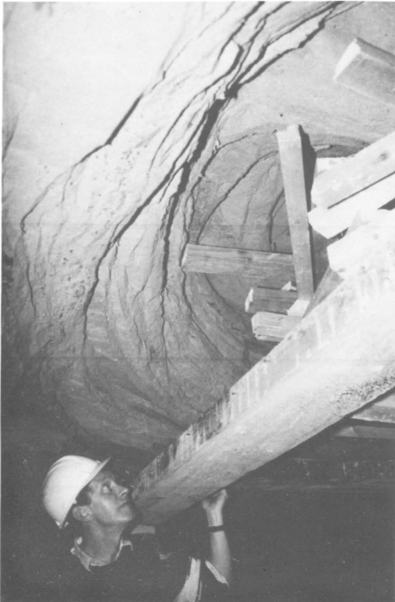
FIG. 6. (above) Saturated sandstone breaking into thin beds and falling away from the roof arch at the southern end of the Stanford Street caves. The light material on the debris pile is fallen roof, some remaining in thin slabs, other broken to sand on impact.
